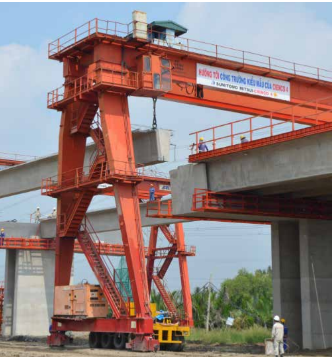
Casting and plunging Super T beams at Tao bridge, Thanh Hoa Province
