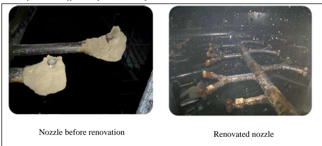
Figure 2.3.12: Nozzle renovation at Iskenderu power plant.
