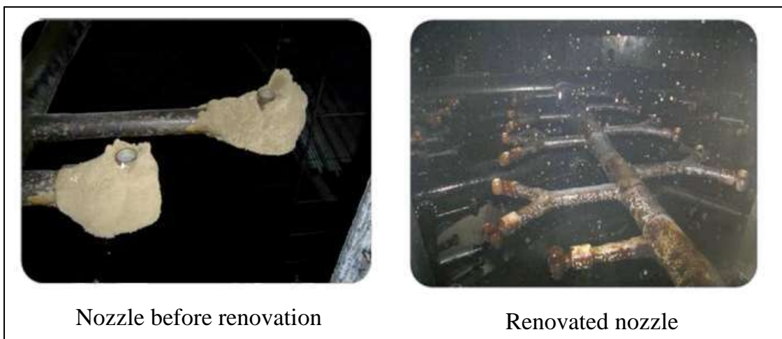
Figure 4.3.17: Nozzle renovation at Iskenderu power plant.
