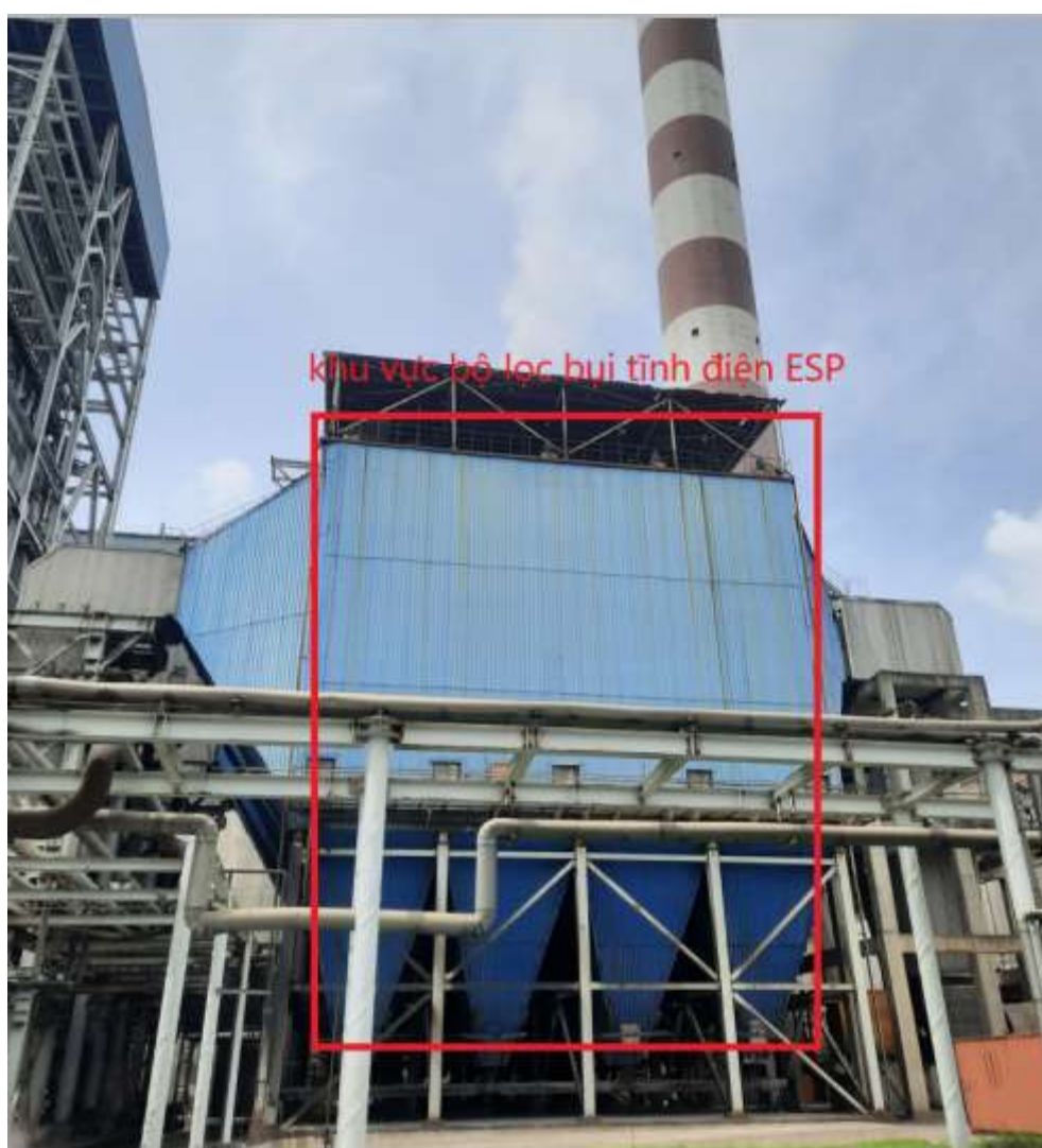
Figure 5.5: Image of the ESP electrostatic precipitator area
